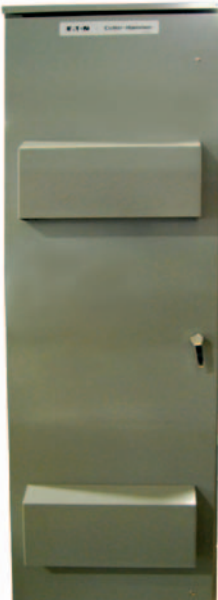
NEMA 3R Drive MCC Section External View
