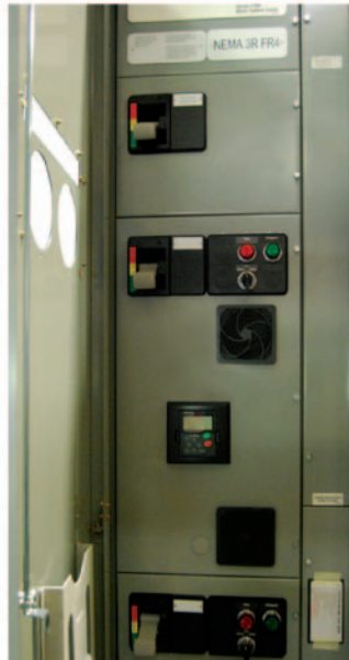
NEMA 3R Drive in MCC Unit Door-Mounted Fans with Filters
